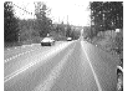
This "before" photo of 228th Avenue show the two-lane rural road design, with no landscaping, no bike or pedestrian facilities, and little management for turning.
