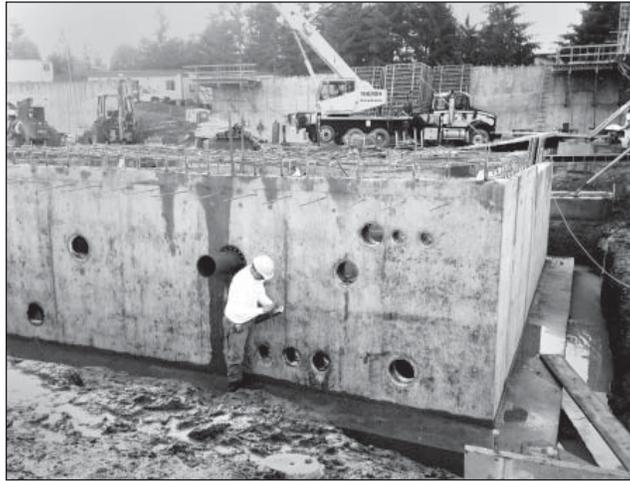
*When a lot of people jump in the pool, the displaced water goes into a surge tank, seen here under construction.*
