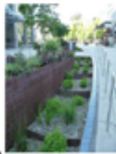
Substantive use of low impact development techniques.
