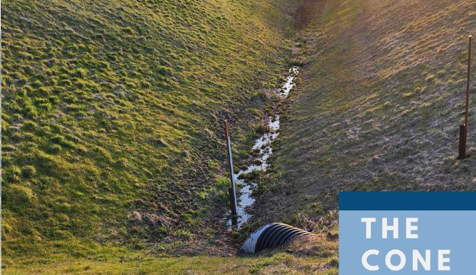
You may notice new equipment in this photo: these are gauges that allow staff to track how high the pond water levels are and help staff respond and prepare for large rain events.
