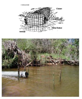
5. *Horizontal Cylindrical Wire Mesh Beaver Guard*: This alternative is used for various sized culverts. There is a large amount of surface area with allows more time between cleanings. It is the simplest design, easily constructible, and low cost.
