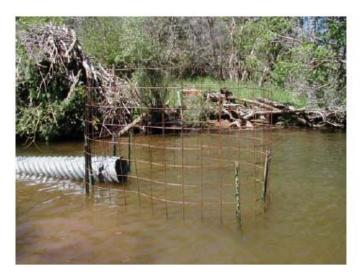
5. **Horizontal Cylindrical Wire Mesh Beaver Guard**: This alternative is used for various sized culverts. There is a large amount of surface area with allows more time between cleanings. It is the simplest design, easily constructible, and low cost.
