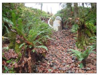
Station 24. Stormwater outfall and energy dissipation structure on right bank of Ebright Creek 4100 feet upstream of Lake Sammamish.
