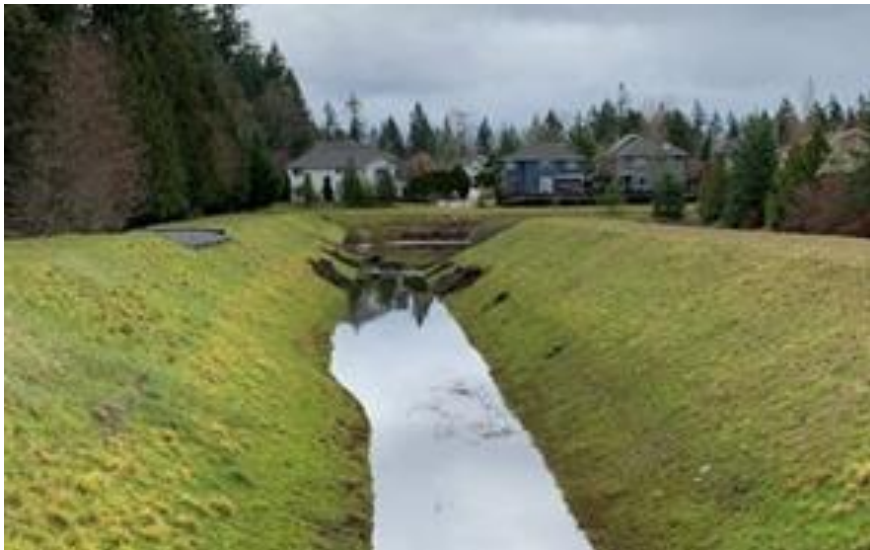
FIGURE 3. EXAMPLE PHOTO FROM A STORMWATER POND WITH RECENTLY COMPLETED IMPROVEMENTS.
