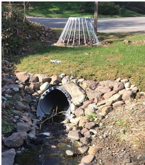
FIGURE 1. NEW CATCH BASIN INSTALLATION AT NE 22ND ST AND 229TH AVE NE
