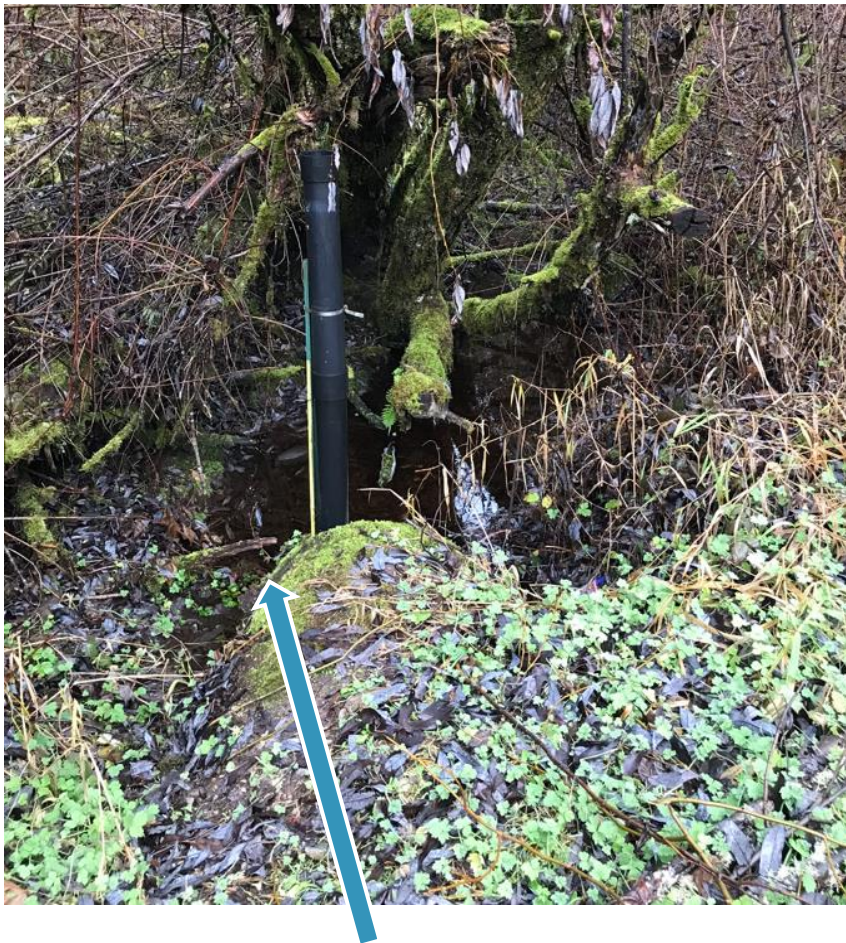
FIGURE 5. HAZEL WOLF CULVERT
